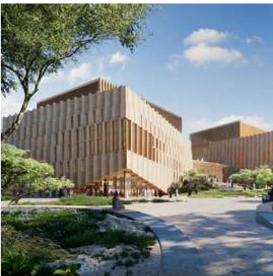
JEDDAH OPERA HOUSE (ONGOING)
